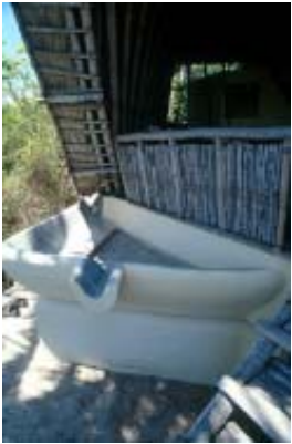
Rainwater filter and overflow
