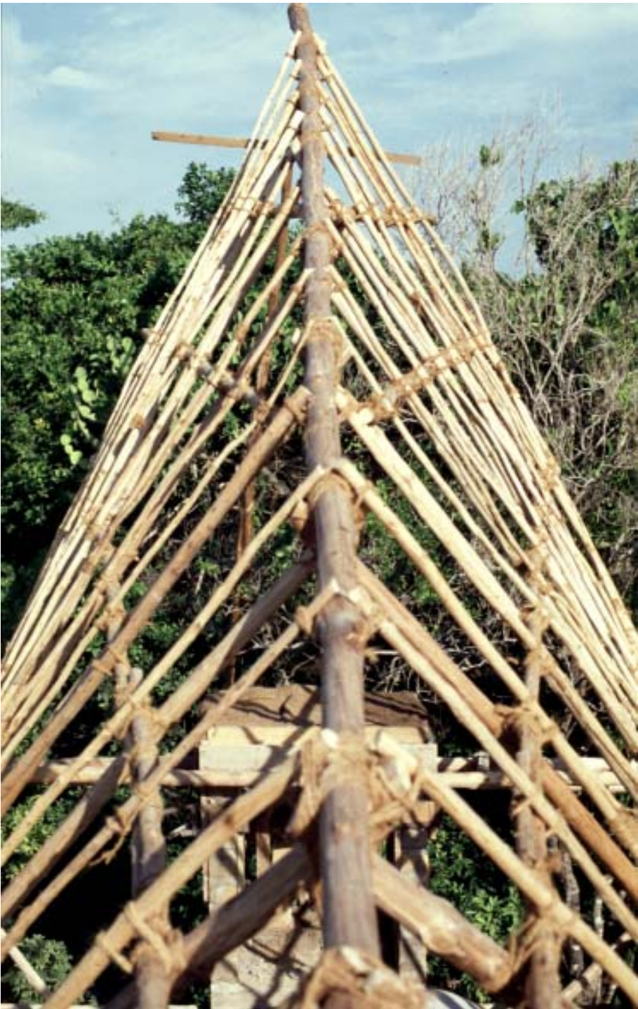
The ridge of the bungalow reaches over the treeline to catch the sea breeze for natural ventilation.
