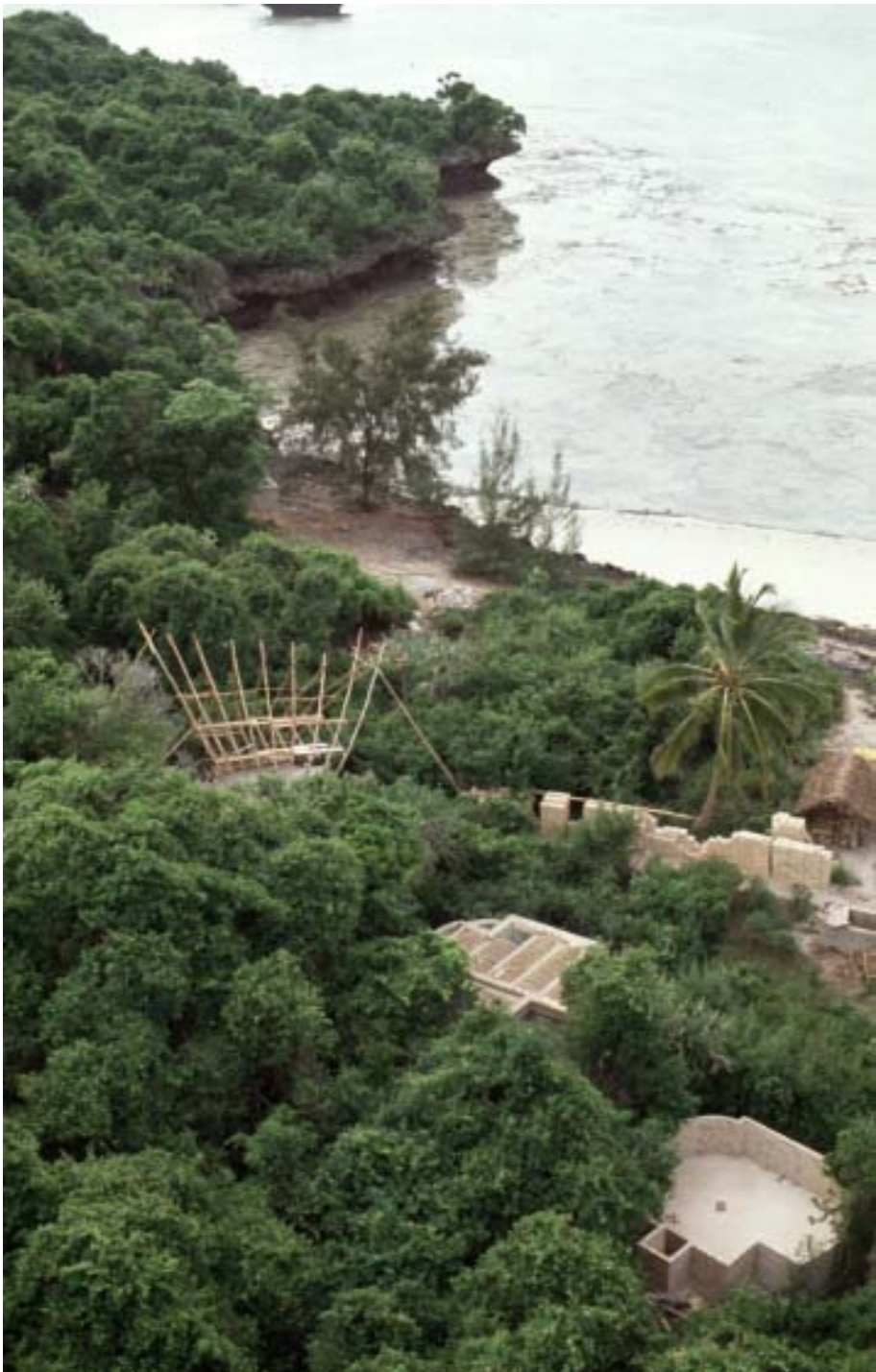
The three building sites, carefully placed into existing openings of the forest, show different building stages: the bottom one shows the cistern's foundation, the middle one the concreted partitions of the cistern and the top one the as yet not covered expressive roofing construction.
