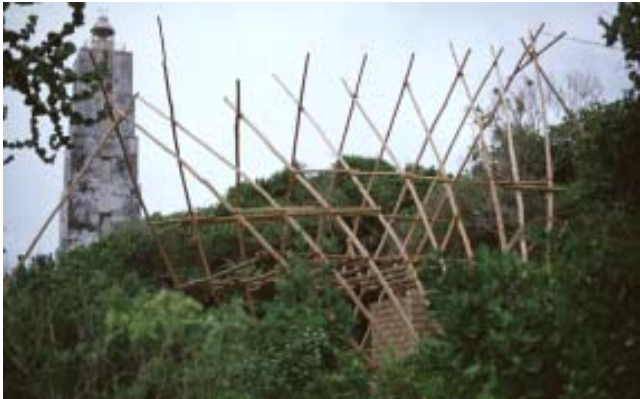
The upright frames are propped up by temporary supporting poles, until ...
