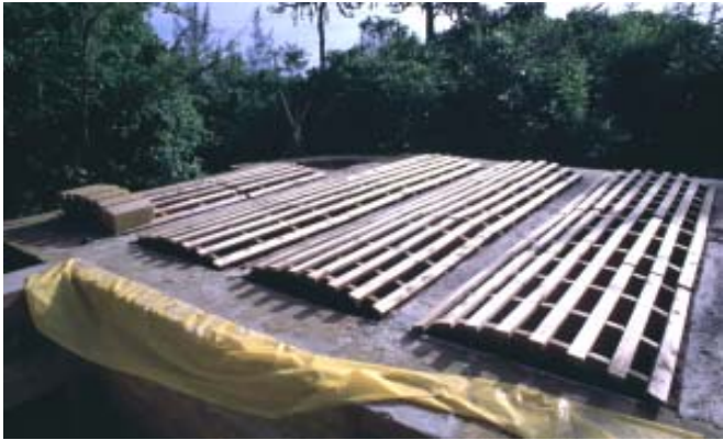
The joints between the sand-cement-blocks, placed on the formwork, will be filled with cement. Once the cement is hardened, the formwork will be removed from the cistern chamber through the revision hatch.
