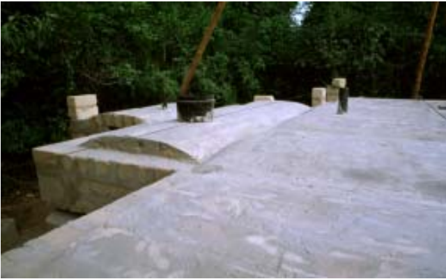
Standard plastic tubes and buckets are used to make openings for water pipes and the compost toilet refuse opening in the vaults.
