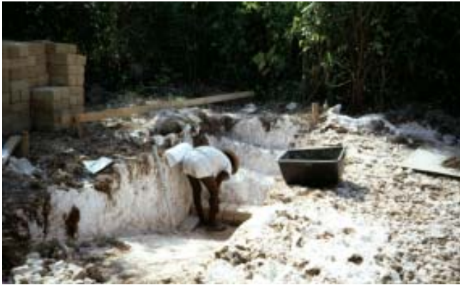
The compost chamber has been excavated from the coral rag. The first blocks of the chamber are laid by Abdi, the foreman.
