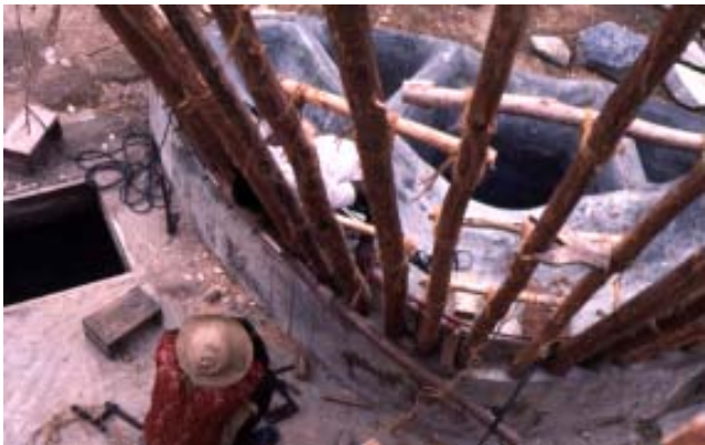
A revision hatch for the cistern is placed close to the filter unit.
