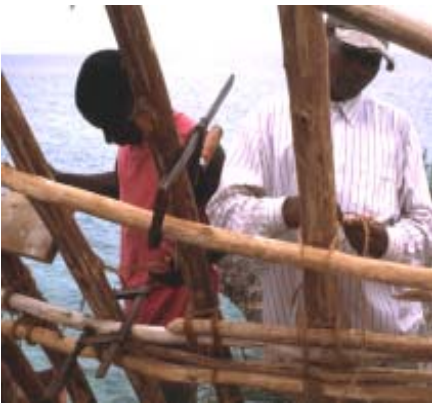
The slender poles from local casuarina-trees are bound together with coconut rope.
