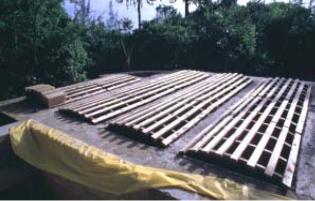
Formwork for the vaulting of the cistern ceiling with bricks in order to avoid the use of easily-corroding reinforcement bars
