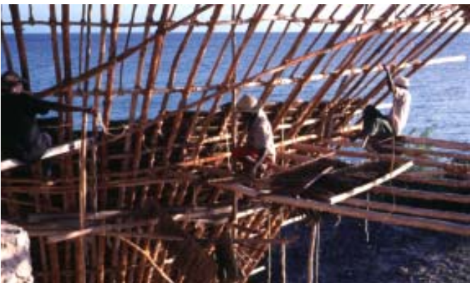
The 'makuti' is placed in horizontal layers, starting from the bottom to the top of the construction.
