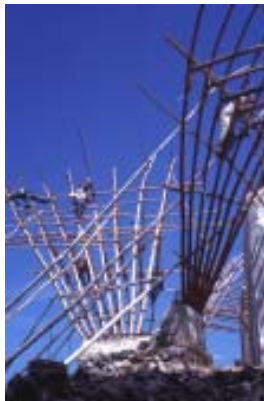
Latticed shell under construction
