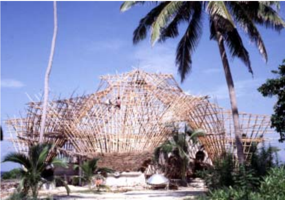
The roof forms a large free-spanning latticed shell construction from slender poles and coconut rope which are bound together with a traditional technique.
