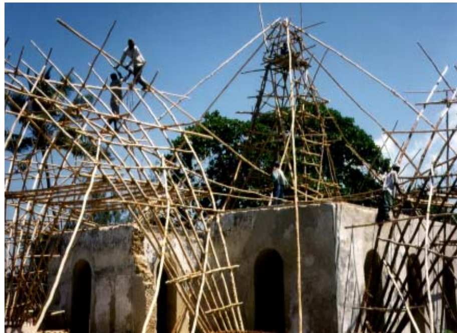
For the construction of the free spanning roof dome of the Visitors' Centre, six latticed shell modules are built simultaneously to meet in the centre of the construction, forming its vertex.
