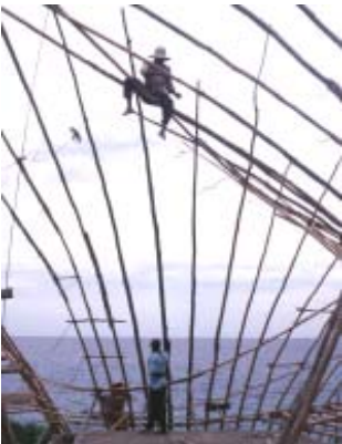
The lattice shell under construction
