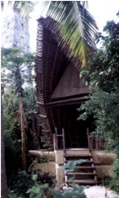
Latticed shell roof on top of the solid base which forms the cistern and rainwater filter
