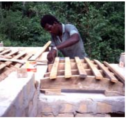
Locally-produced cement earth bricks were used for the solid base which holds the cistern
