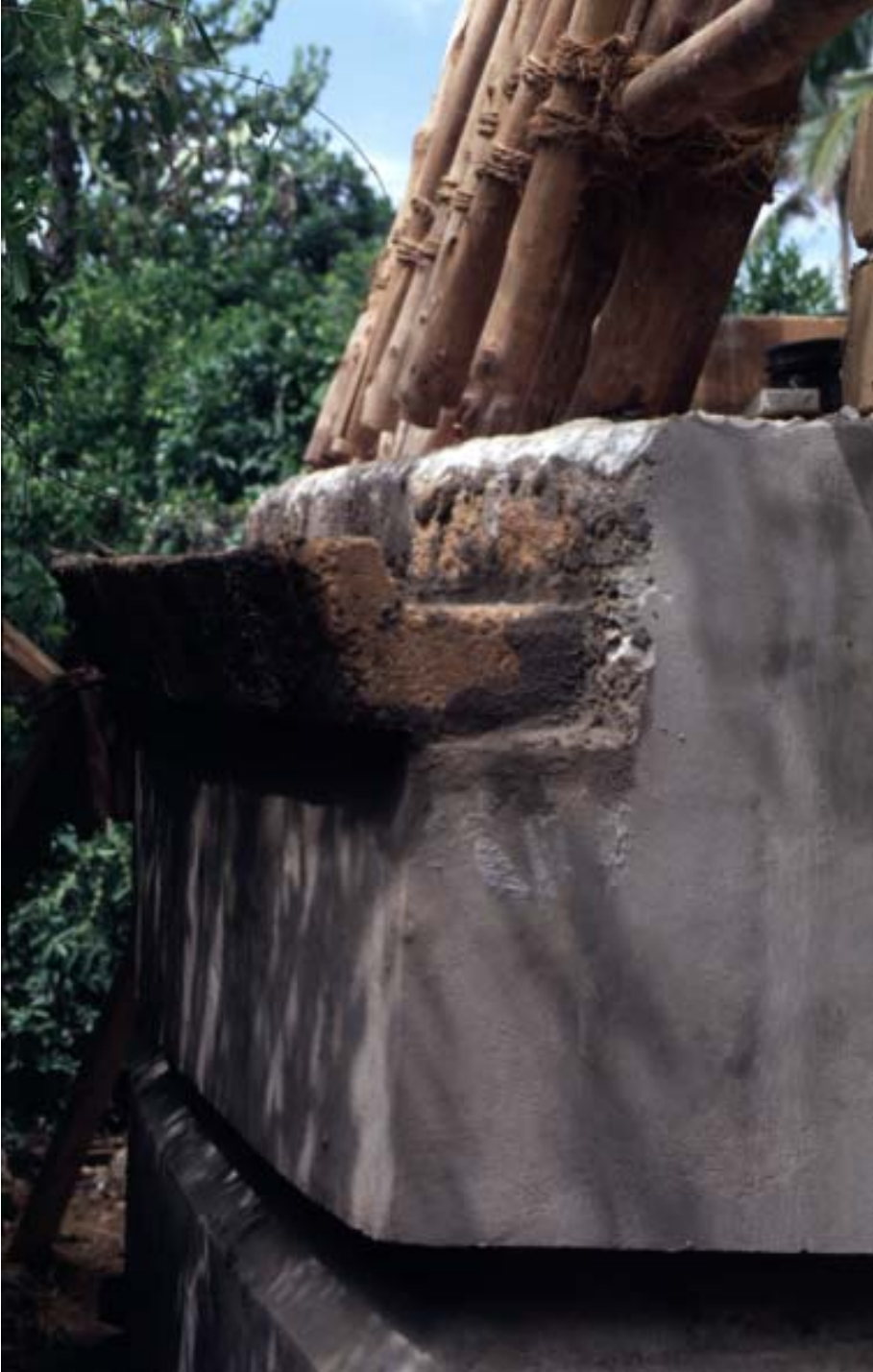
The rain water gutter below the footing points of the roof frames is wide enough to collect tropical rains. The groove running around the base of the bungalow is a measure to prevent termites from entering the house.
