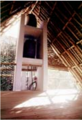
'Technic Tower' with hot and cold water tanks, solar power system
