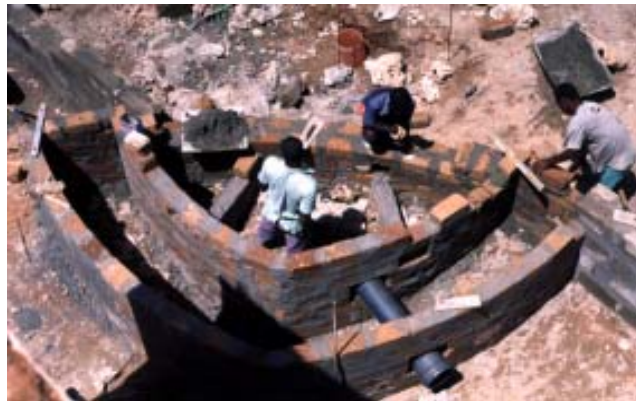
A 'filter and foul flush' unit, which also forms a footing point of the roof dome,
