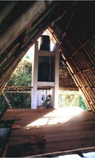
'Technic Tower' at the rear of the bungalow with hot and cold water tanks and space for solar batteries.
