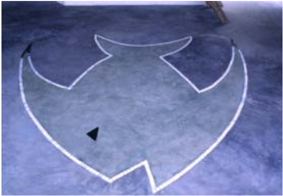
The floor is made from coloured cement decorated with marine motives
