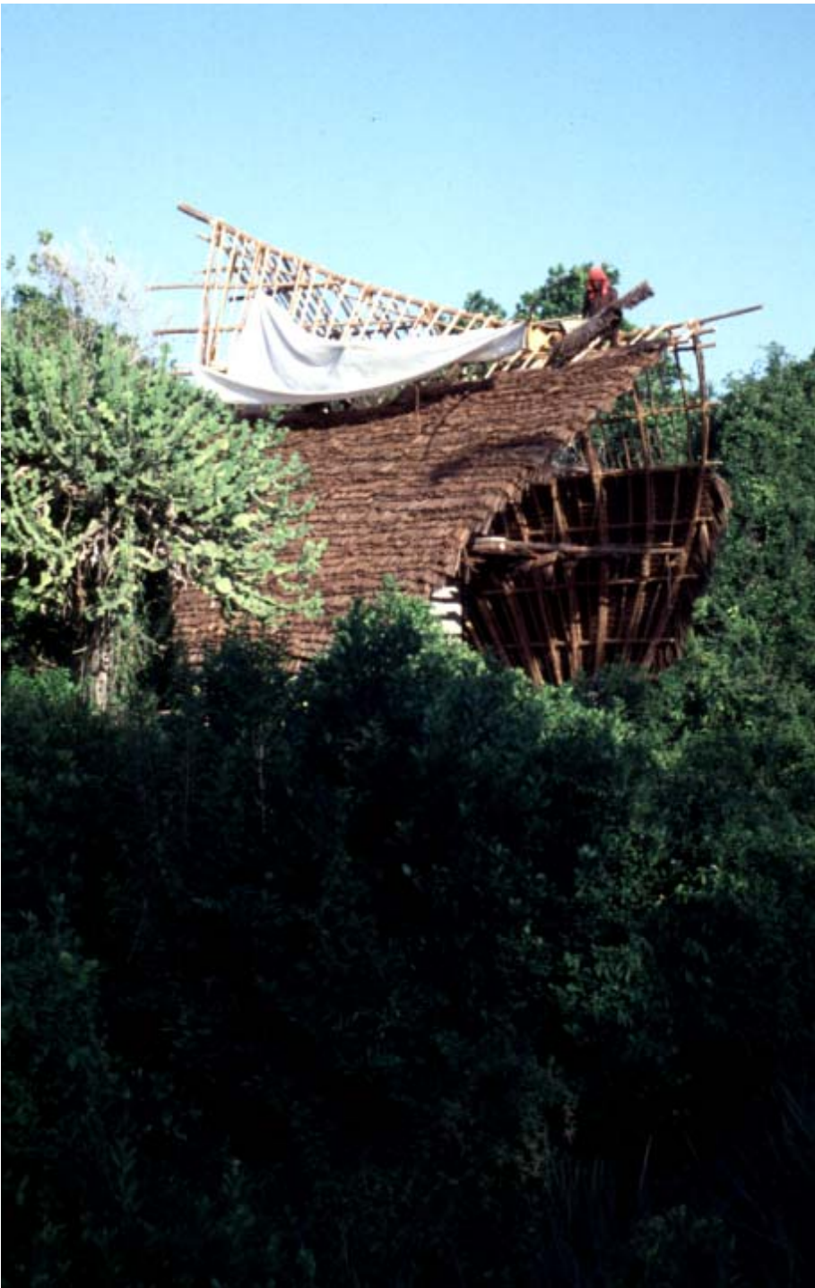
The roof is nearly covered on both sides with 'makuti', the local roofing material made from coconut palm trees.
