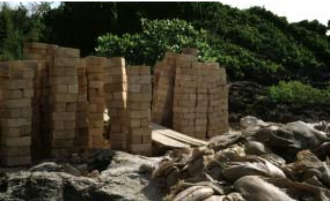
Sand and aggregates packed in bags, and blocks from Zanzibar are deposited above the high tide water mark before being taken to the building sites.
