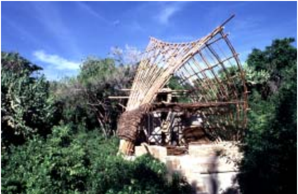
The latticed shell construction forms a pliable, but very stable structure.
