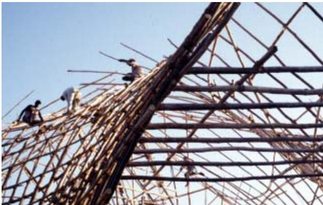
One latticed shell module under construction.
