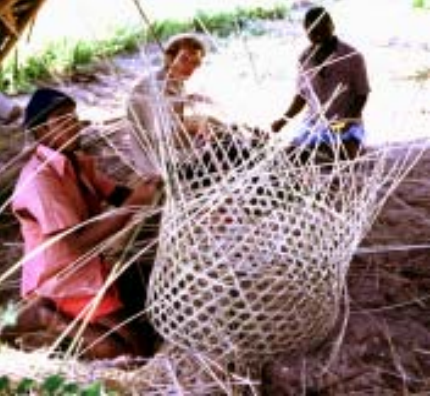
Weaving of 'madema' from reeds for partitions
