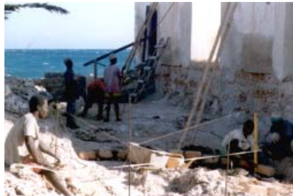
At the base of the former lighthouse keepers' house cisterns are excavated to store rain water.
