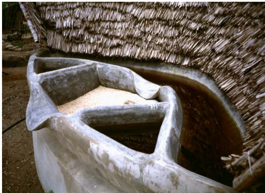
A 'filter and foul flush unit' in use. According to the prevailing water level, the water flows into the next partition.
