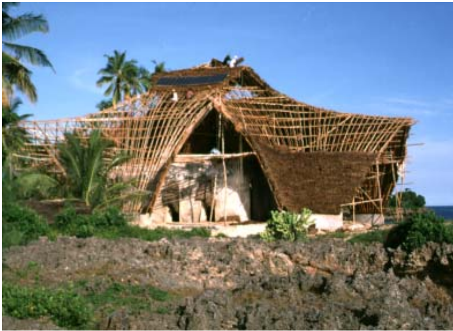
The roof dome is partly covered with 'makuti'. Solar panels are installed to provide energy for lighting and radio communication to Zanzibar.
