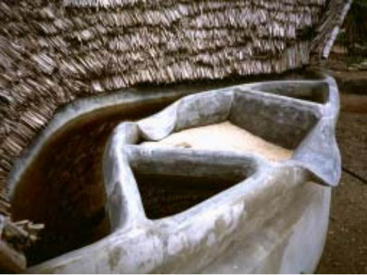
Rainwater gutter and filter and 'foul-flush' basin of the Visitors' Centre
