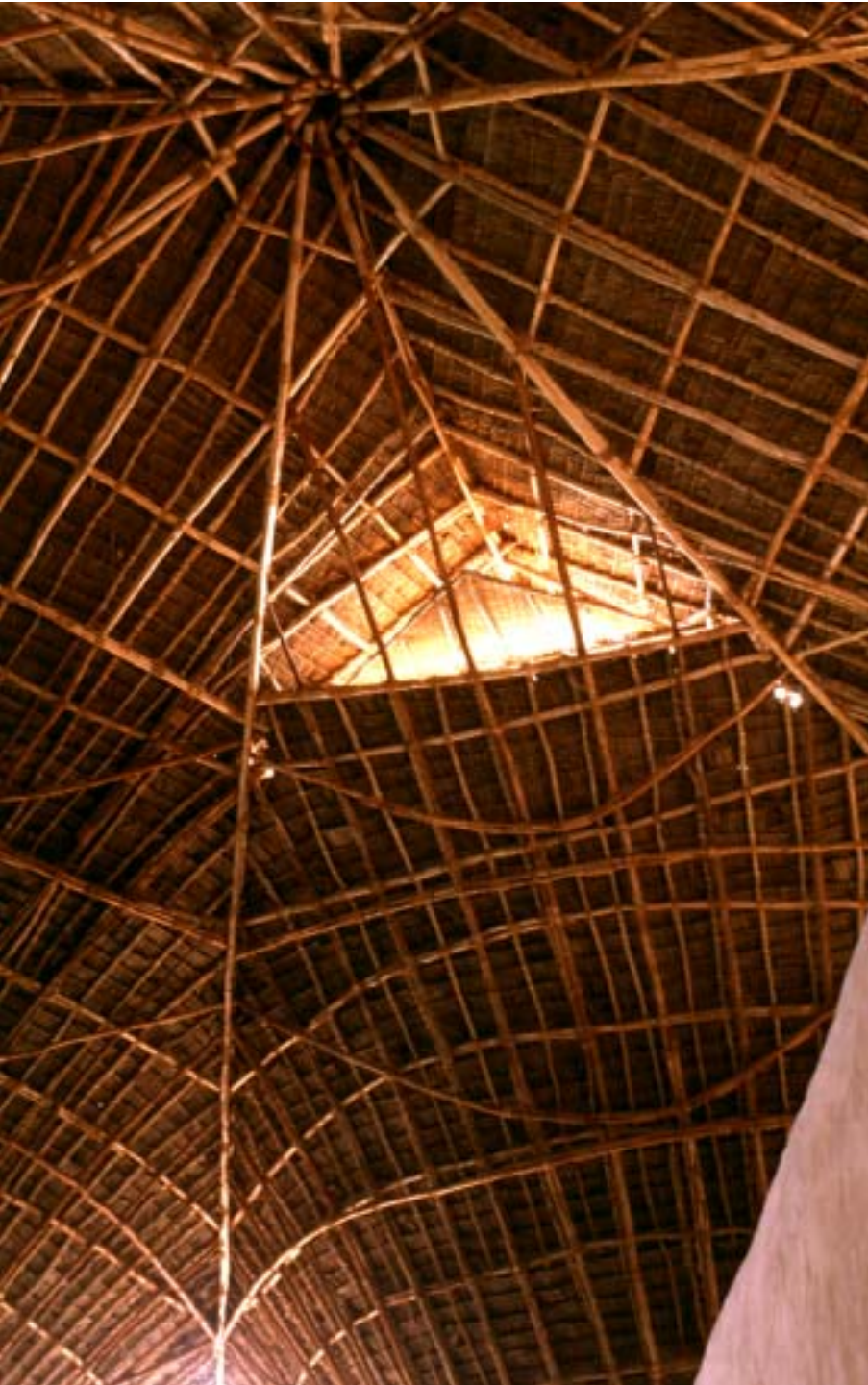
View of the vertex and a skylight of the roof dome.
