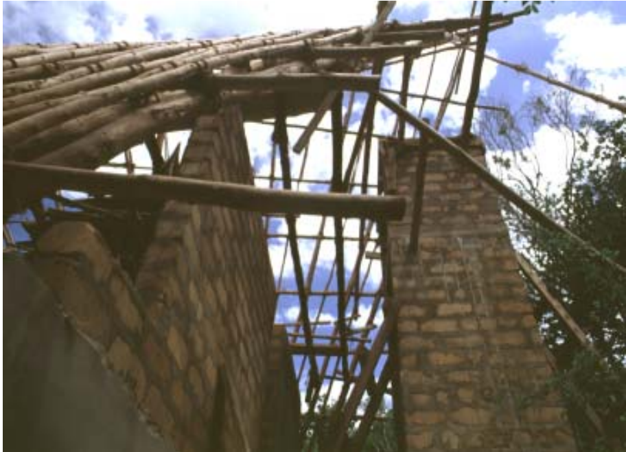
In contrast to the solid 'technique tower' and the partition wall to the bathroom, which are made from blocks, the light roof is made from local poles.
