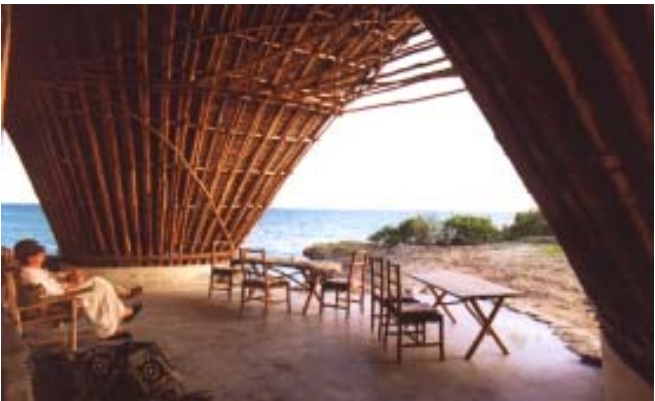
The Western terrace of the Visitors' Centre facing seawards, showing the footing point of the dome.
