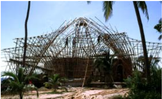
The dome of the Visitors' Center under construction. The dome is probably the biggest free-spanning dome made from slender poles and coconut ropes.
