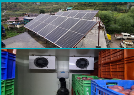
Figure 6: An 8 MT Cold Store powered by an 8 KW Solar PV System at Andhra Village, Shimla District
