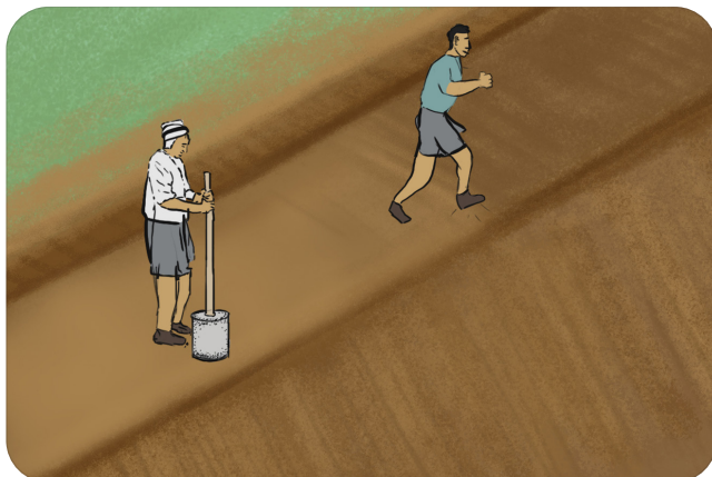
Dike compaction process done manually
