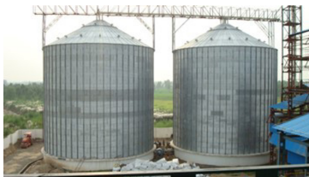
Figure 3.2 Grain Storage Silo
