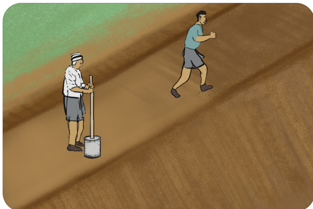
Dike compaction process done manually
