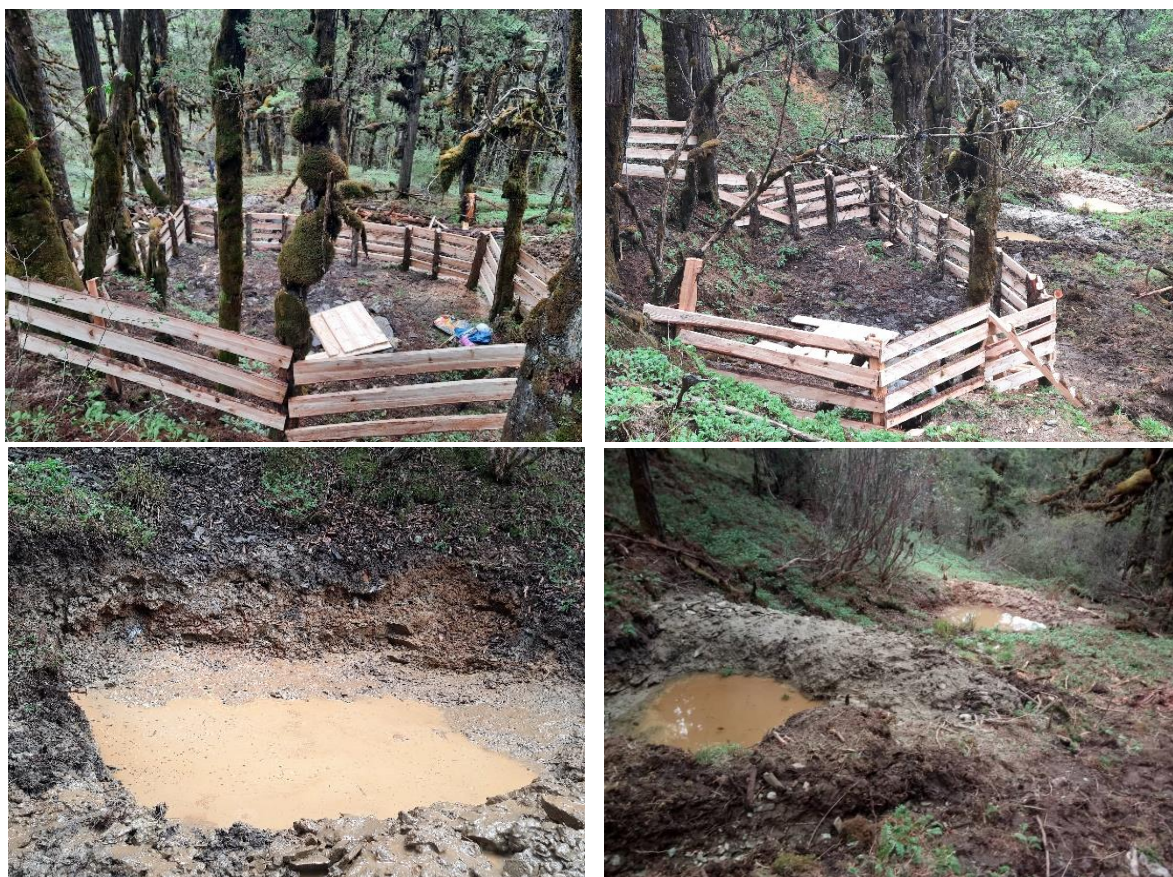
Photo: After work completion
