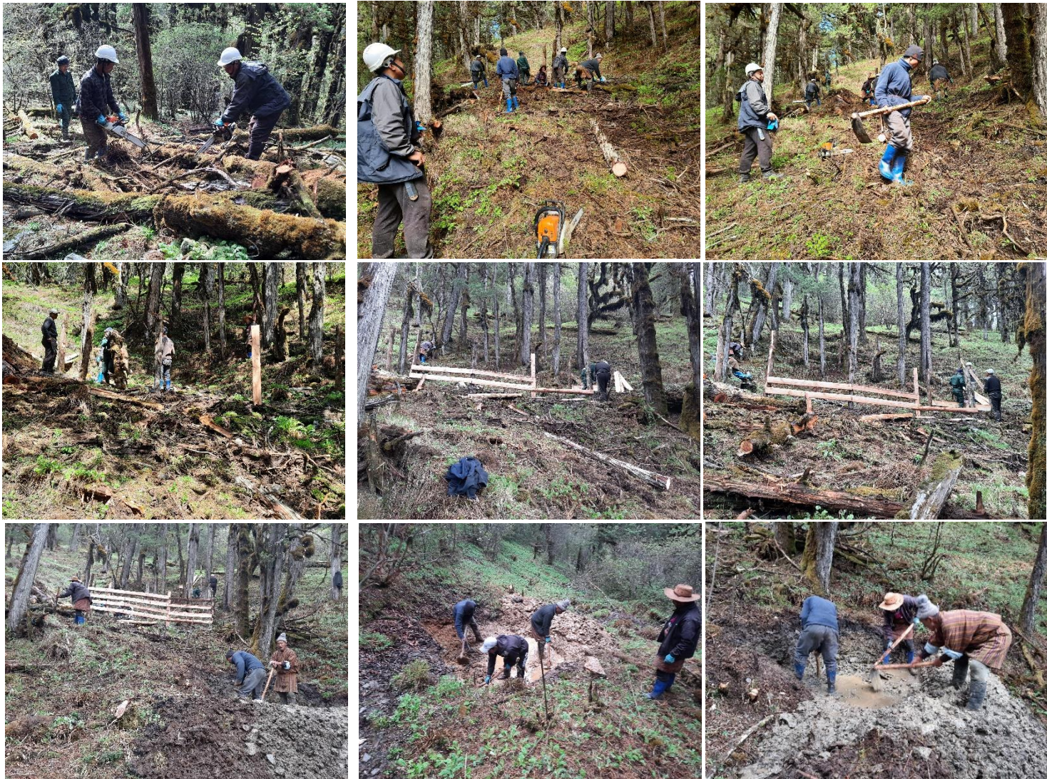
Photo: Work execution
