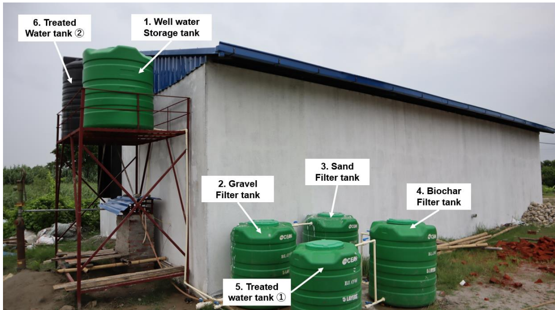
Figure 35. Process water treatment system
