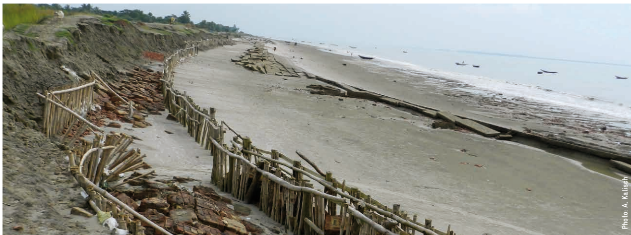
Eroding embankment on Mousuni Island
