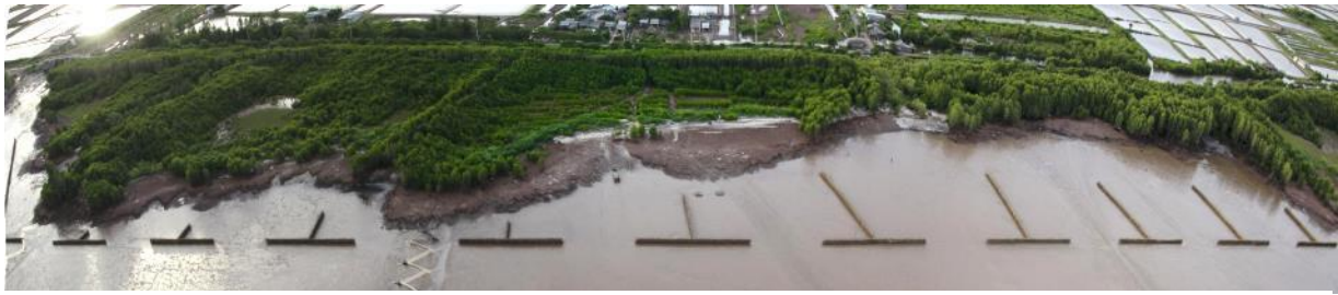
The north-eastern coast of Bac Lieu Province: The breakwaters reduce wave power and trigger sedimentation for future rehabilitation. Barren, saline land between the coast and the dyke is being rehabilitated and the hinterland is protected.
