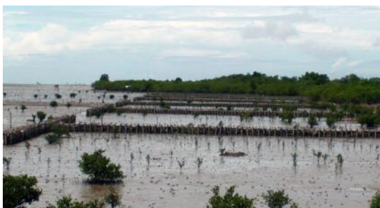
Mangrove rehabilitation between bamboo breakwaters in Vinh Trach Dong, Bac Lieu.
