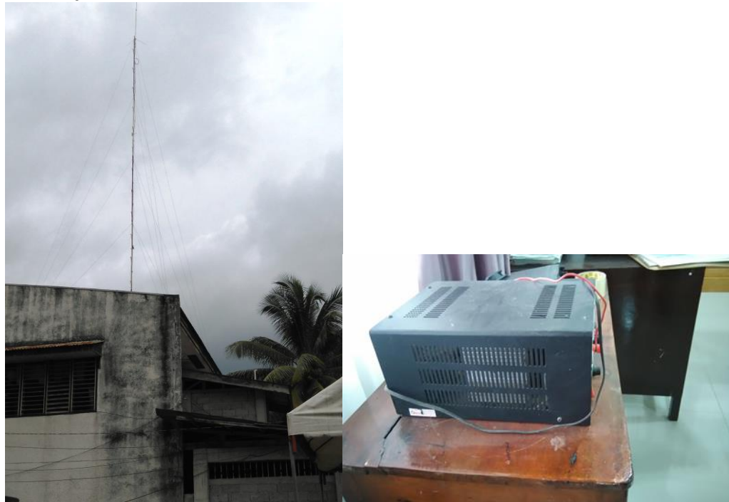
The radio & communications system connecting Maasin with its neighboring municipalities
