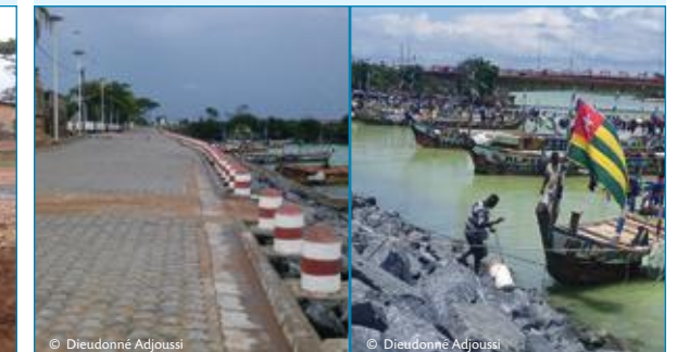
Protective structure on the southern shore of Lake Togo and fishing boats moored against the new bank
