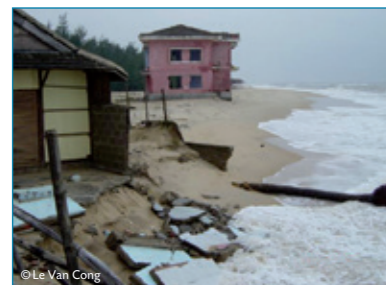
Coastal erosion in Vietnam
