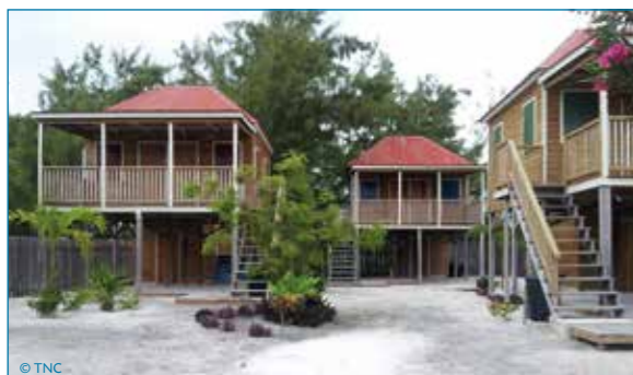
Building on stilts may reduce vulnerability of infrastructure
