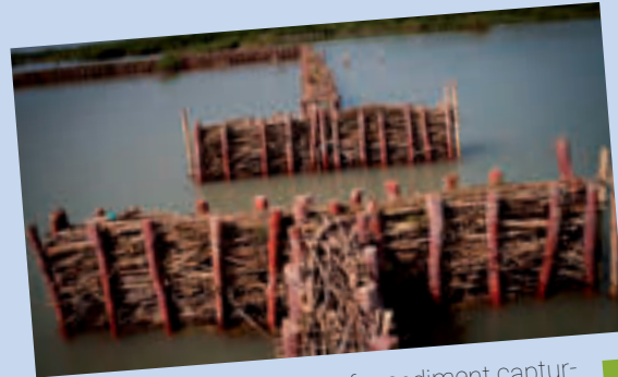
Permeable dam structures for sediment capturing © Nanang Sujana
