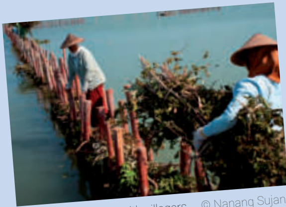
Permeable dam structures for sediment capturing © Nanang Sujana
