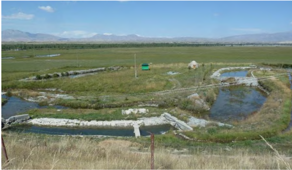
Fig. 7 Water dam facility NE of Bash-Kaiyndy N of the hay fields at the position lat: 41.163749, long: 75.926079 (Source: own image P1010524.jpg from 09/04/2015).
