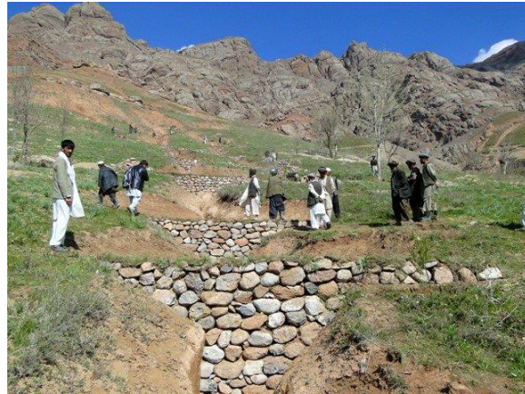
Figure 7: Gully treatment with stone barriers. Left: scheme from Studer and Liniger 19 . Right: photo from Afghanistan (Source: WOCAT ).
