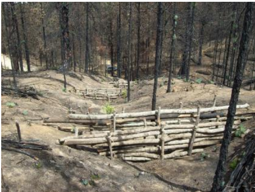
Figure 8: Example of gullies treatment with wood barriers.
