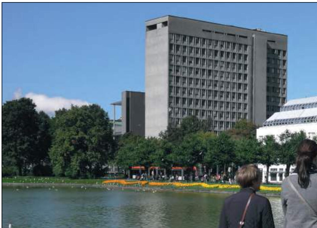
Figure 9.3 Rehabilitation of Bergen City Hall.
