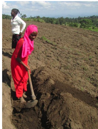
Measuring and digging of contours prior to establishing contour bunds
