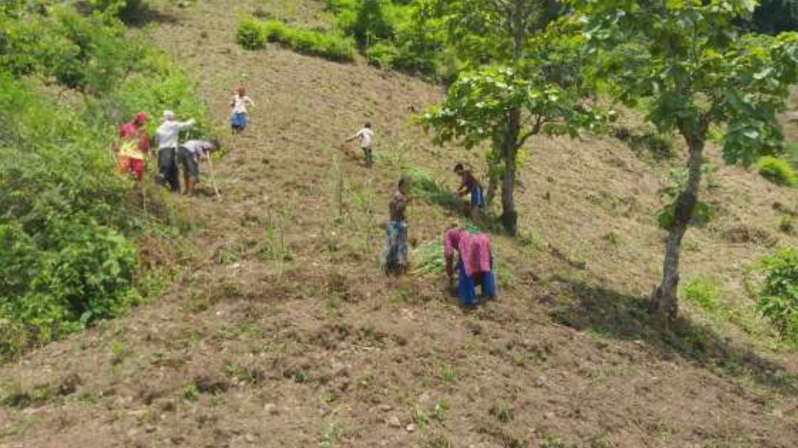
Plantation of broom grass on landslide prone cliffs
