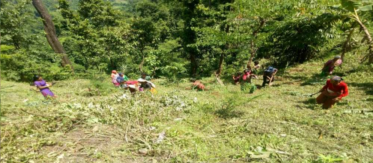
Plantation of broom grass on landslide prone cliffs
